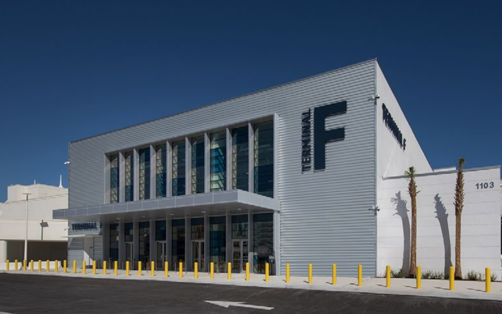
PortMiami Terminal F Renovations – Miami, FL
