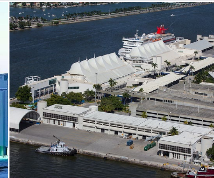
PortMiami Command & Control Center (C3) – Miami, FL
