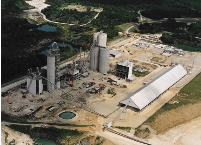
Thompson S Baker Cement Plant - Newberry, FL (Courtesy of VP Buildings)
