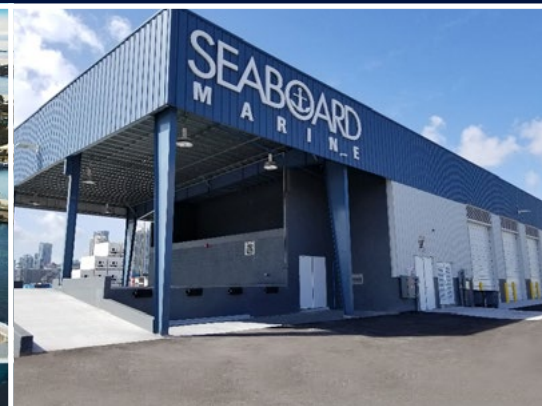
Seaboard Maintenance & Office Building – Miami, FL
