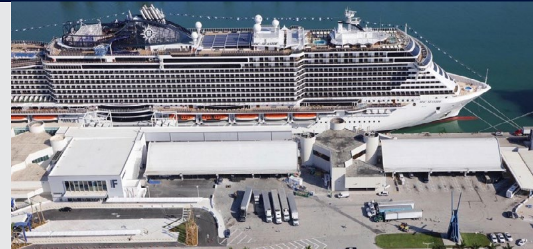
PortMiami Terminal F Renovations – Miami, FL
