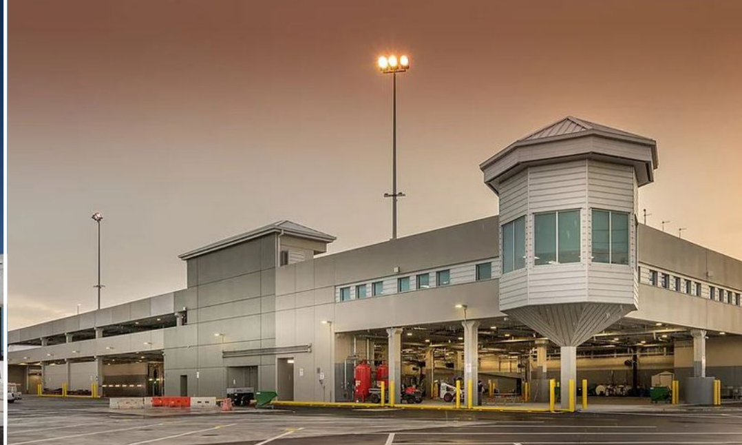
Ravenswood Bus Maintenance Facility – Dania Beach, FL
